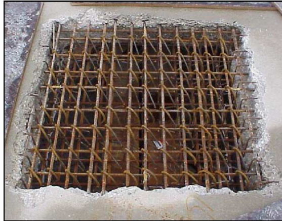
Fig. 8. Slab reinforcements after hydro-demolition.
